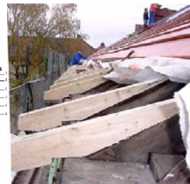
▲ Roof overhang for future insulation
