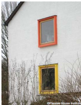
▲ Placement of windows for future wall insulation
